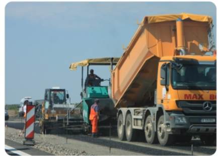
Facility Emergency Repairing
